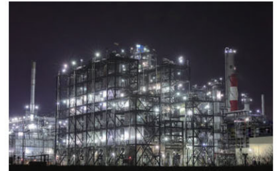
Suitable for lighting in chemical factory
